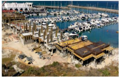
engineers designed a 500 mm deep raft foundation for the load bearing walls to replace pilings or standard strip footing. The use of Crystal Admix
